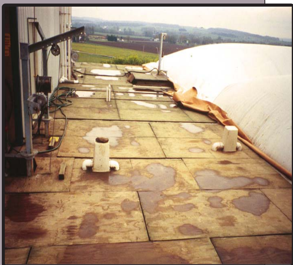
Influent, food waste and effluent pits covered by plywood
