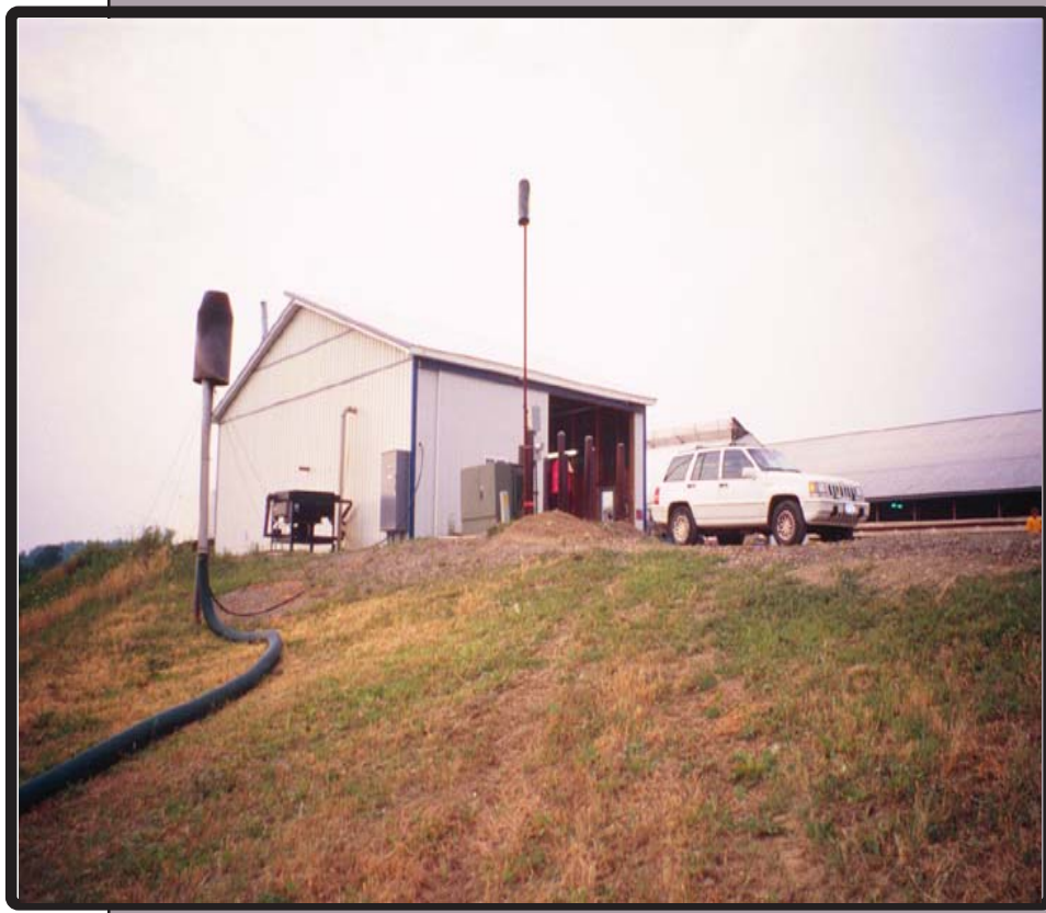
Gas utilization building with flare to left
