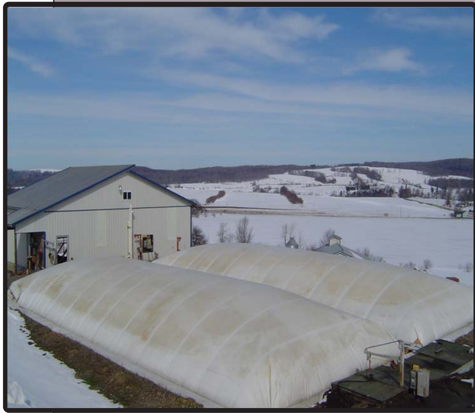
Twin digesters with separator building in background
