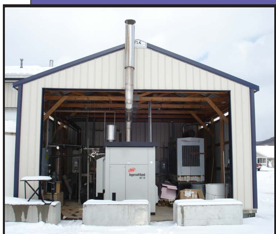
Gas utilization building
