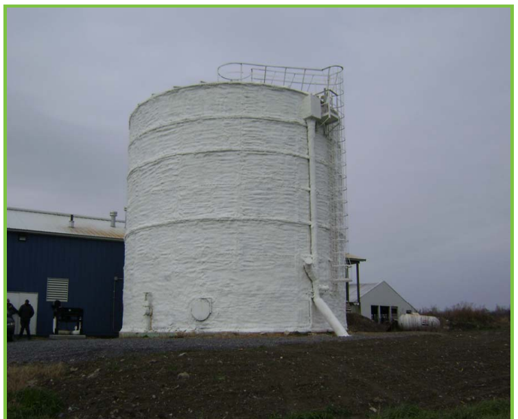
Sheland Farm's complete mixed vertical anaerobic digester
